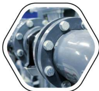
PIPE FLANGE JOINT
